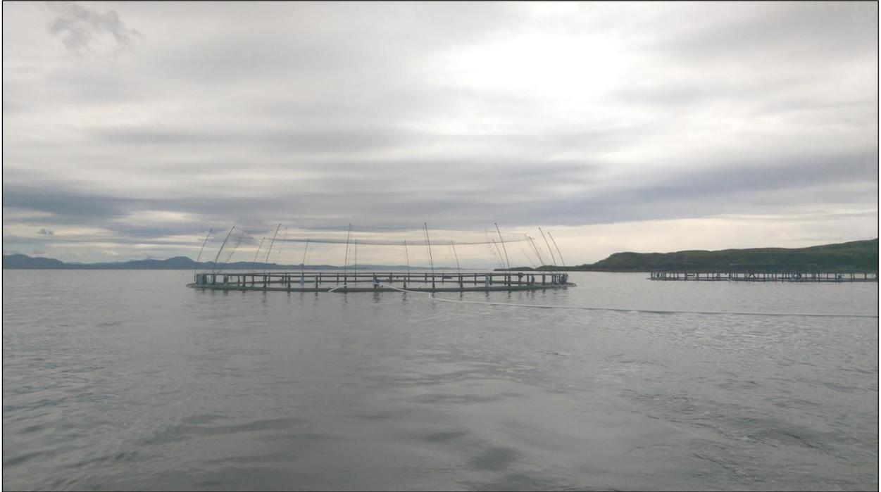
*Figure 2: Typical pen design measuring 120m in circumference. This shows poles at the perimeter of the pen which support the top/bird netting and white pipes delivering the feed from the barge.*
