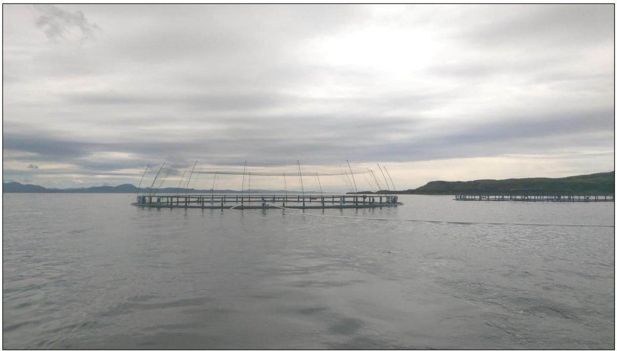
*Figure 2: Typical pen design measuring 120m in circumference. This shows poles at the perimeter of the pen which support the top/bird netting and white pipes delivering the feed from the barge.*
